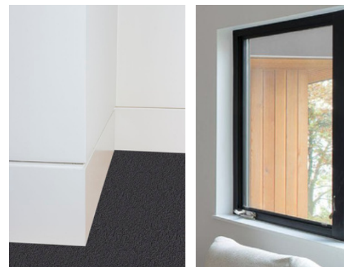
FLUSH BASEBOARD DETAIL DRYWALL RETURN WINDOWS & DOORS MAIN FLOOR
